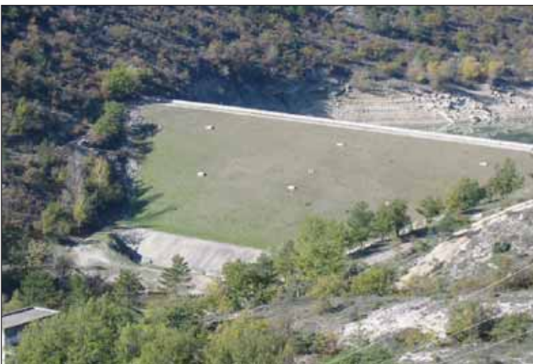
Downstream view of La Laye dam in France.
