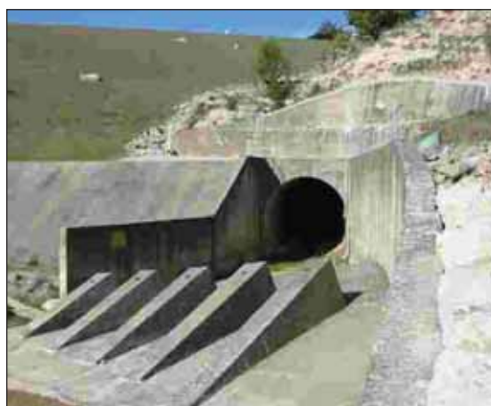
The spillway outlet.
