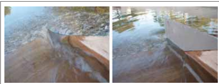
Inlet of the sill before and after the flow optimisation (1000 year flood).
